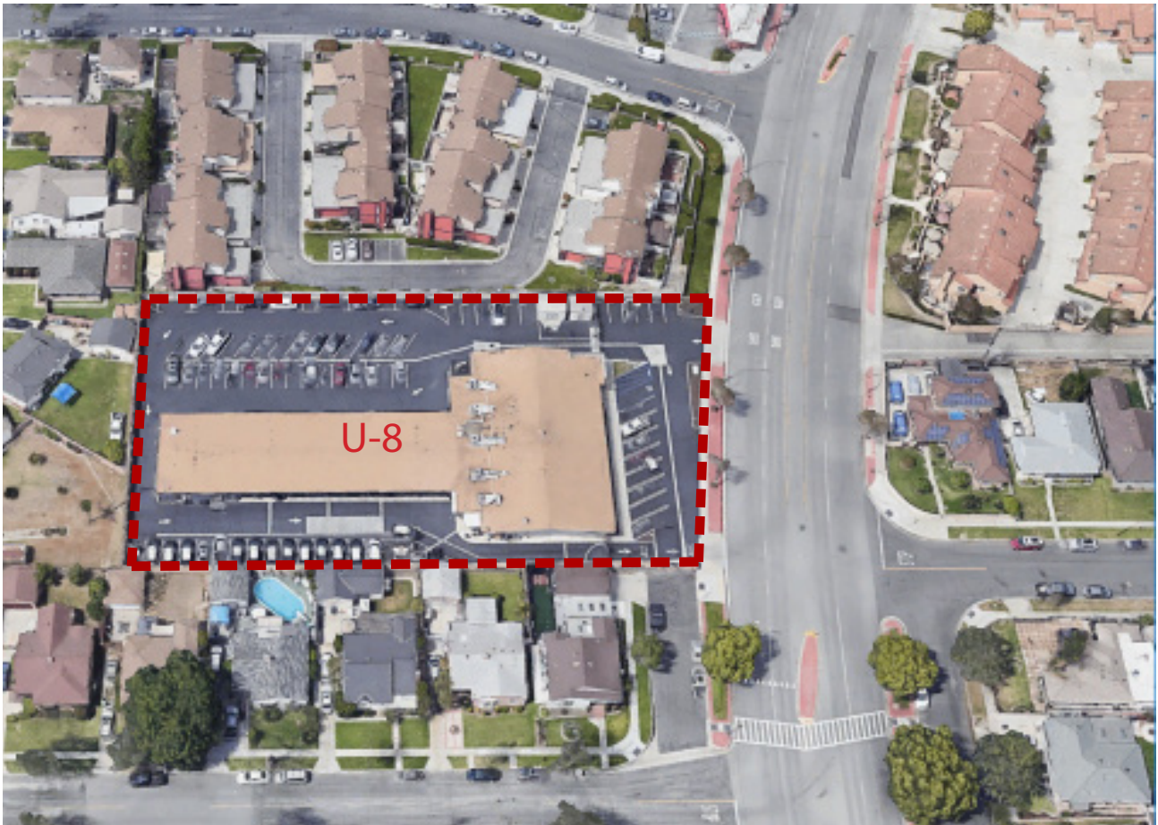
Site U-8: California Highway Patrol Site
